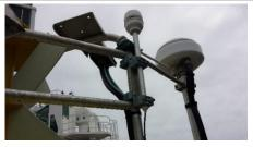
**Comment from PI:** The meteorological station is mounted at the top of the BOREL superstructure. There is no central data storage available on the buoy.
